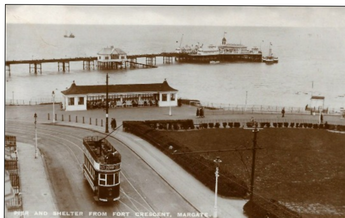
An early postcard showing the original Fort Crescent Public Shelter with a paddle-steamer at the end of the Pier (or Jetty) in the background and an electric tram in the foreground
