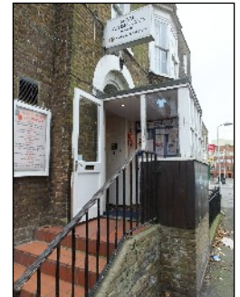
Right: The steps leading to the storm-porch at the entrance to Legion House
