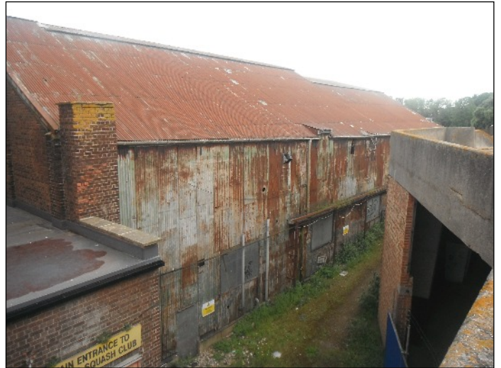
One of the former hangers from Westgate RNAS now behind Dreamland Ballroom (This photo was taken from the roof of the Arlington Centre in June 2013)
